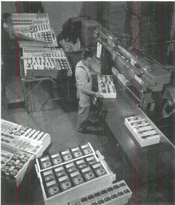
CENTER, LEFT. Stripping a combination label form. Stripping is done by an automatic electric precision cutter. By one easy push of a button, the form is moved into position and cut—a single automatic machine operation. In the background is one of several automatic lifts and jogging tables, which enable the cutting-machine operator to double his production.
